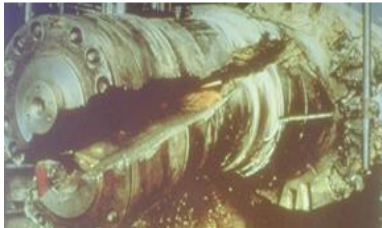
Figure 2 — Cracked Power Plant Rotor
